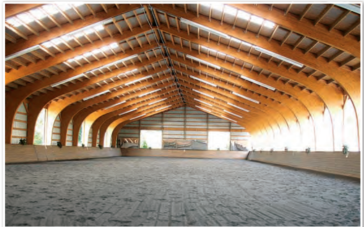
72'-0" Span • 16'-6" Eave • 6.75" Width • Staunton, VA
