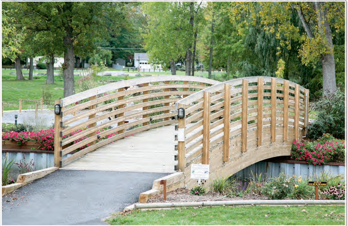
8' x 58' • Pedestrian Bridge • Livonia, NY
